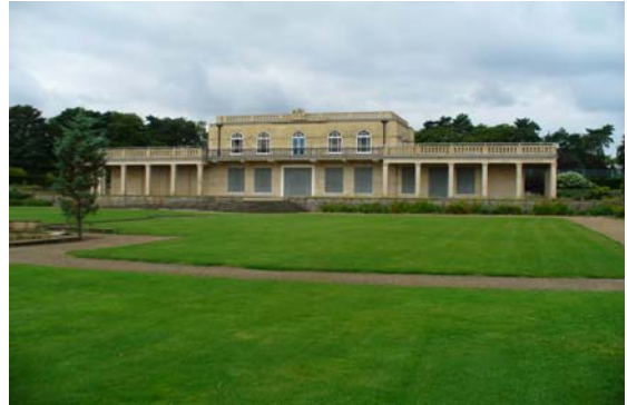
Waterloo Park Pavilion
